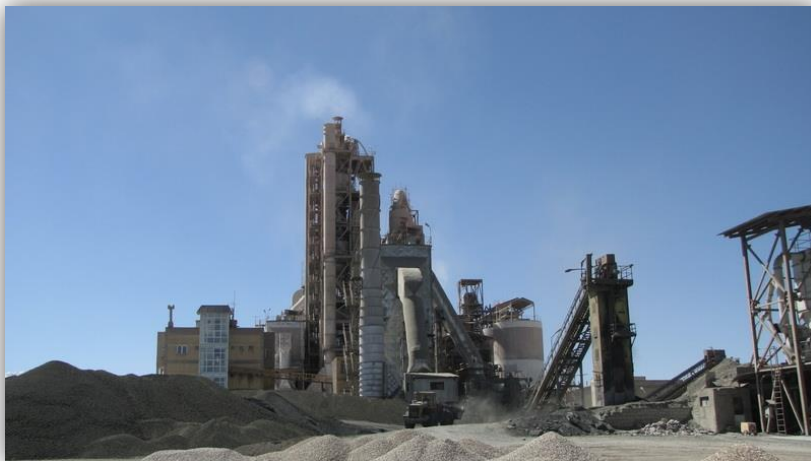
Abadeh Cement Factory
