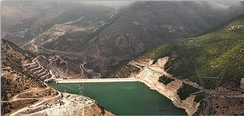
Siah Bishe Pumped Storage Power Plant
